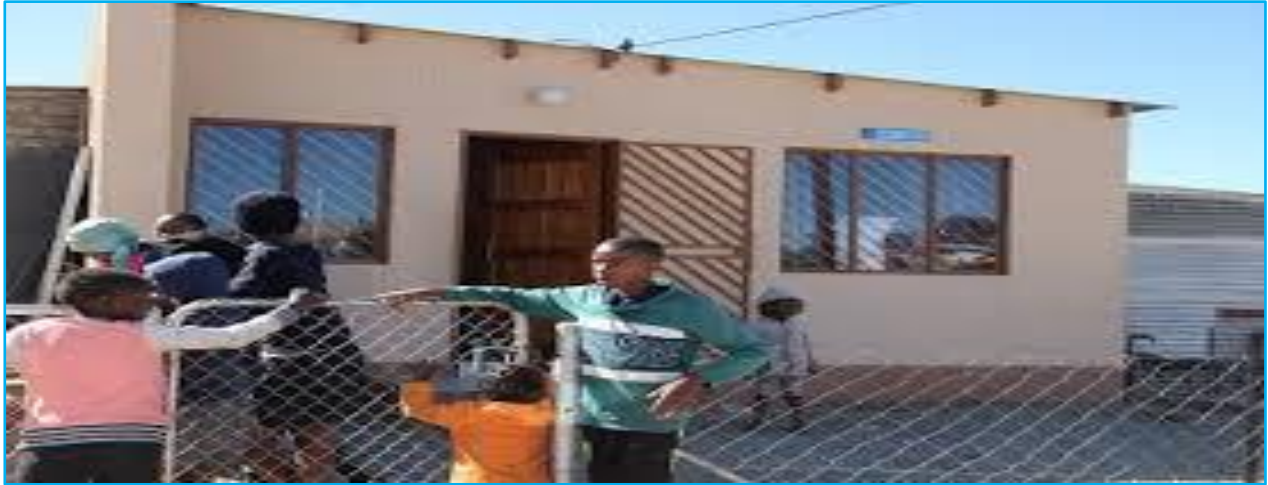
Figure 14: picture of a house built under the informal settlement upgrade program.
